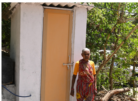
Retrofitting of individual household toilet
